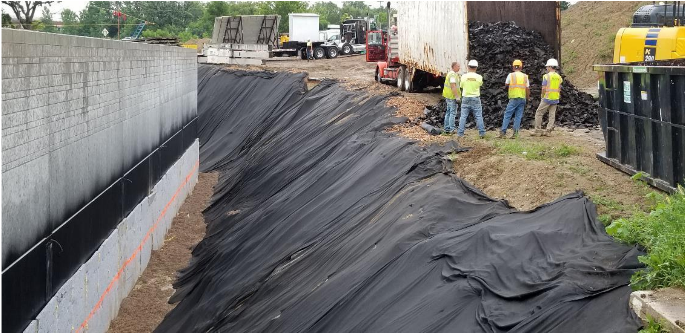
TDA is placed in 2-foot lifts
